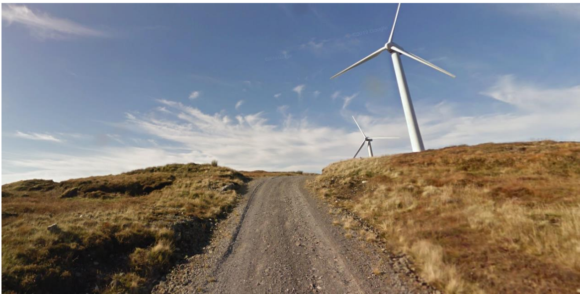
Photo 3: Road leading to T21 proposed to be decommissioned and restored
